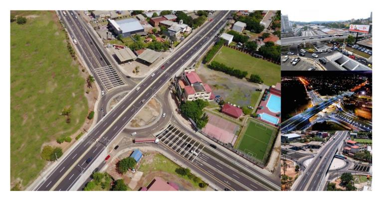
The project is a grade separation consisting of a bridge and a tunnel, which have completely changed the traffic flow at the intersection between Madame Lynch St and Aviadores St, removed the existing congestion and improved general traffic flow in Asuncion city.
